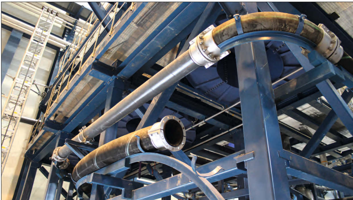
Installation of Slurry Hose System.
